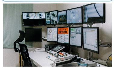
A networked control system that manages production, shipment and quality is mounted, enabling quick and efficient daily operation of complex compounding calculation as well as massive amount of forms processing on paperless basis.
